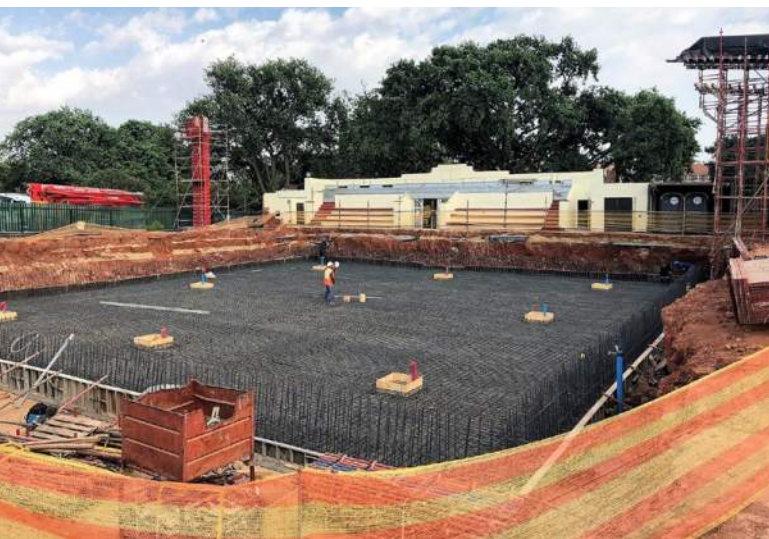
Large pool base reinforcement and first western roof column cast (courtesy of WCSE)
