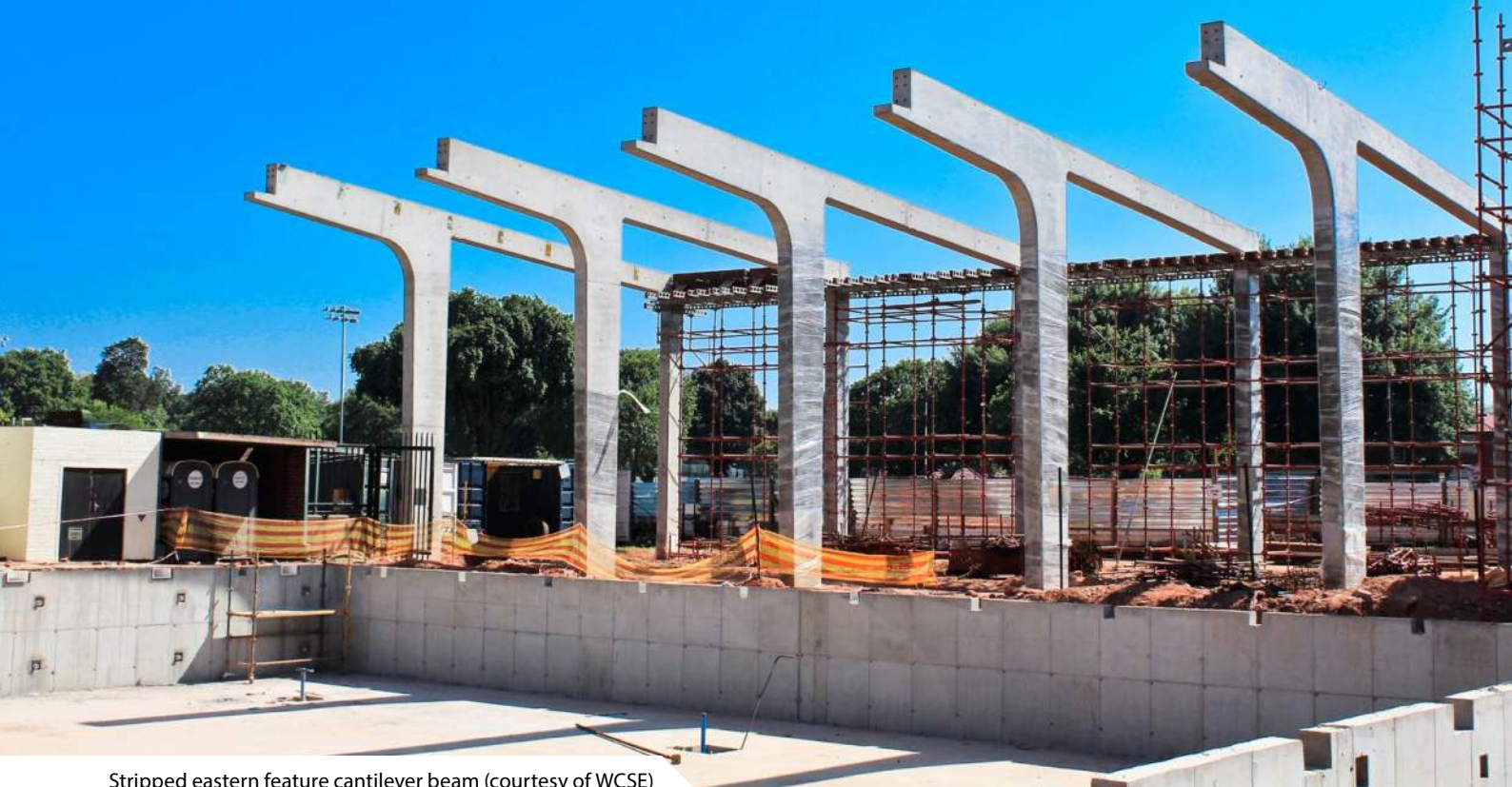
Stripped eastern feature cantilever beam (courtesy of WCSE)
